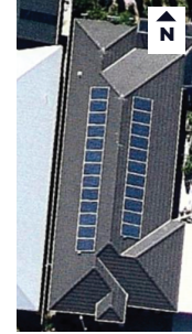
3.025kW East : 11 Panels 3.575kW West : 13 Panels
